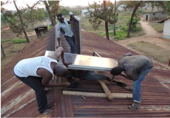
Technicians at Chilala-Focal Development Colleges (FDC) in Lindi installing solar panels donated by SATF.
